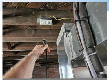
Major – condensate pump is not plugged in. Condensate drain line does not terminate outside
