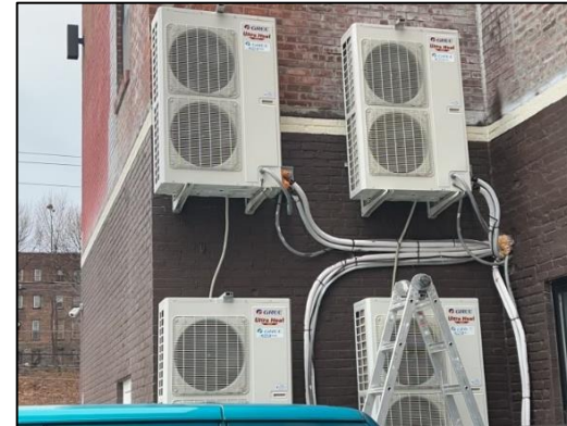
Same-day repair: diversion hoses
